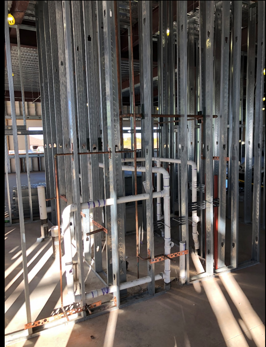
Gymnasium Face Brick, Interior Framing and Plumbing Rough-in
